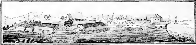
A view of the Lines thrown up on BOSTON NECK by the Ministerial Army. 1. Boston. 2. Mr. Hancock's house. 3. Enemy's camp on M o Hill. 4. Blockhouse. 5. Guardhouse. 6. Gate & Drawbridge. 7. Beacon Hill.
